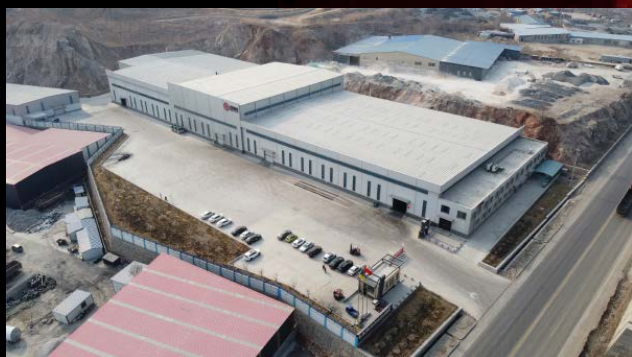
Plant 1. Magnesia Carbon Bricks, EBT Tap Hole Bricks Manufacturing Unit
